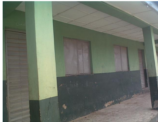
Plate 5: Block of class-rooms donated to Sepeteri community
