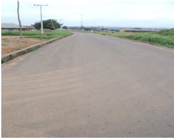
Plate 3a: Road development in Sepeteri community
