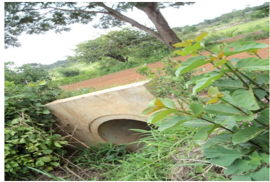
Plate 4: Drainage and culvert construction in Ogundiran community
